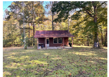
Cabin with covered porch
